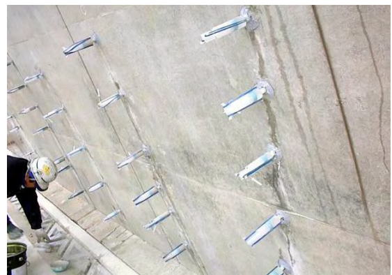
ひび割れ補修（低圧注入）状況：橋脚
